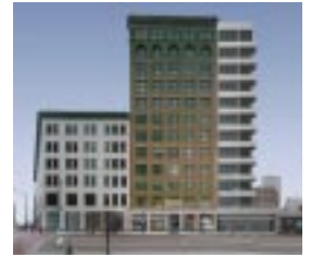
145 High Street, Courtesy of Long & Wilcox
