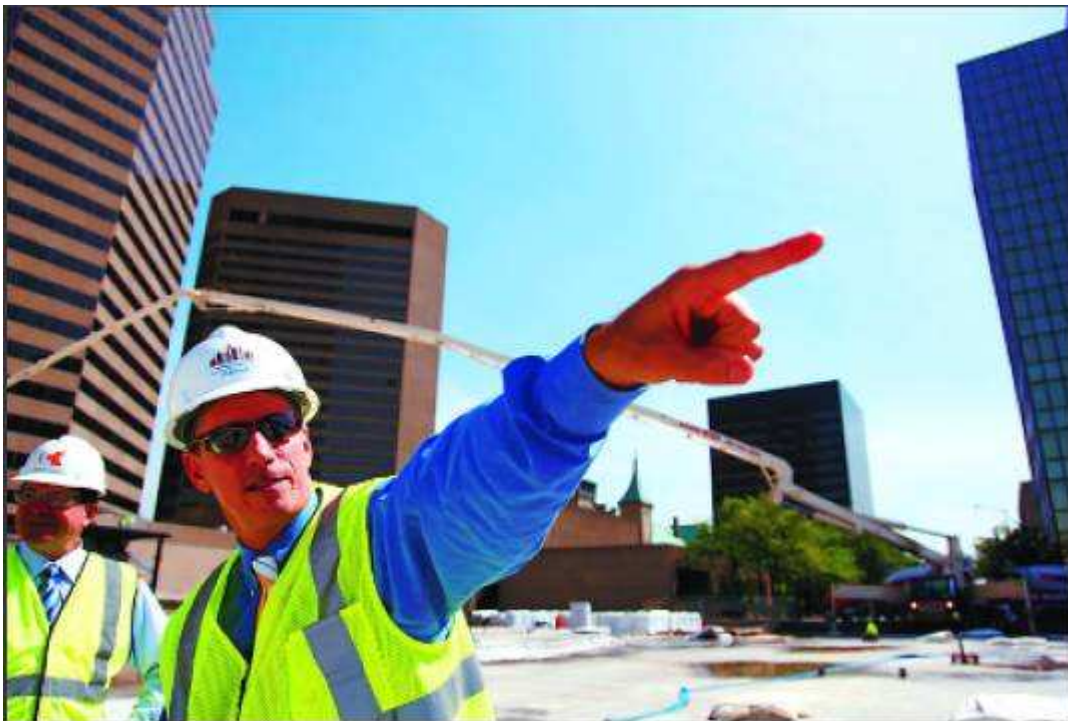
Guy Worley, president and CEO of Columbus Downtown Development Corp., with contractor Mark Corna behind him, points out features at the site.
